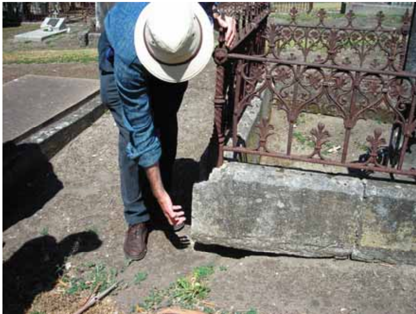
Inadequate drainage undermining foundation stones
