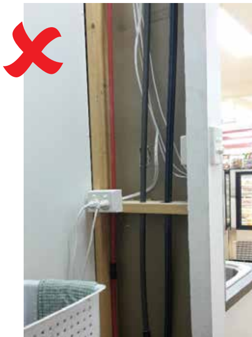
Non-complying - wall cannot be effectively cleaned as not smooth and impervious.
