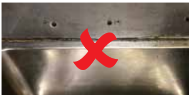
Non-complying - gap between basin and splashback.
