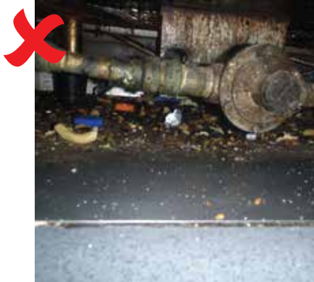
Non-complying - not able to be cleaned effectively.
