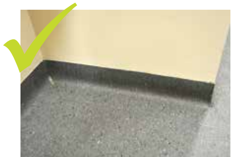
Complying - floor coving.
