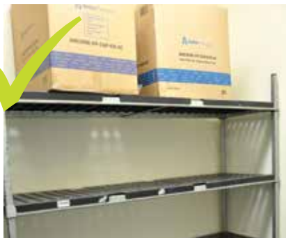
Complying - shelving which is in good repair, smooth and impervious.
