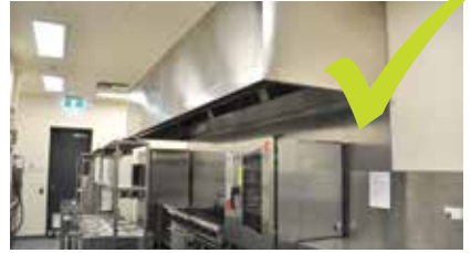
Complying - lighting with shatter-proof covers.
