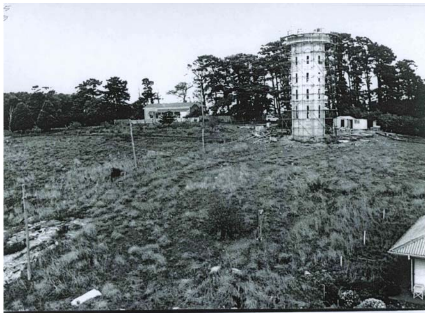
View from the hospital to the south of the Nurseryman's Cottage and the Water Tower under construction in 1959.
