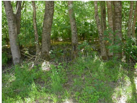
Detail of stone retaining wall on lake margin. Note the line of the wall between the trees and marked by the differential ground heights.
