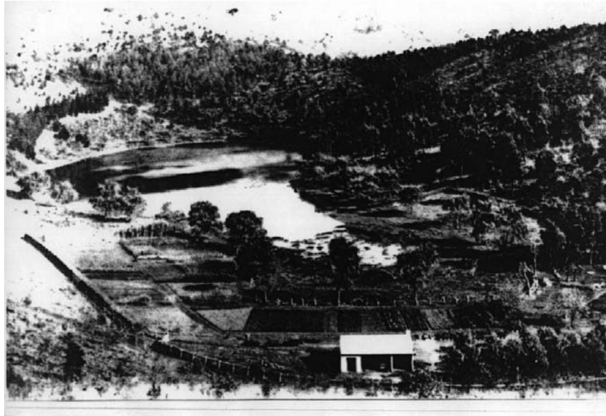
View of Leg of Mutton Lake to the south c.1885. Note that the Nurseryman's Site Shed in the foreground is open to the north.
