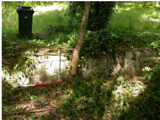
Centre east-west wall at east end showing wall height and construction and split level nature of building.
