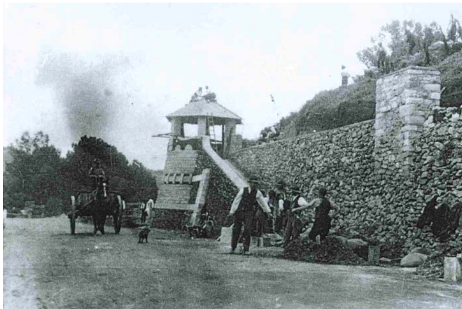
Working bee on the Blue Lake Embankment, 1918 (Source: Les Hill Collection )
