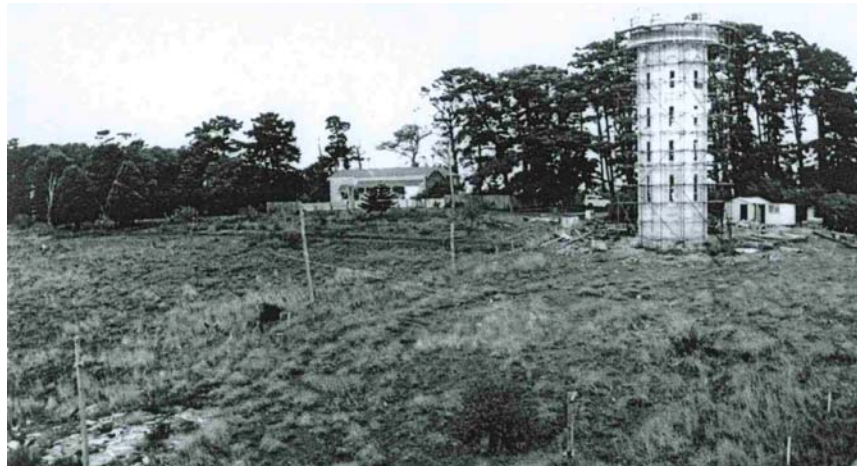
The Nurseryman's 'good stone cottage' in 1959, with the water tower under construction. (Source: Les Hill Collection)
