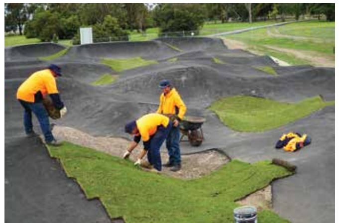
Pump Track construction at Hastings Cunningham Reserve.
