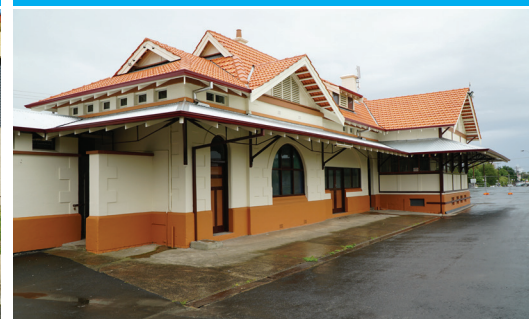
Railway Station external restoration
