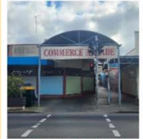
3 Commerce Arcade and Ripley Arcade laneway entrances
