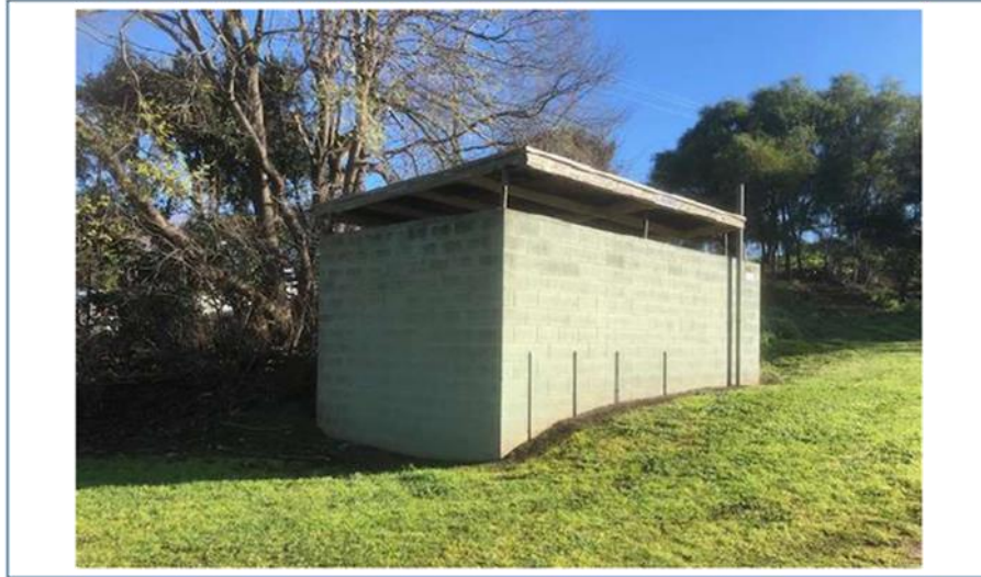
Fig: 5. Toilet block at North side of the club building
