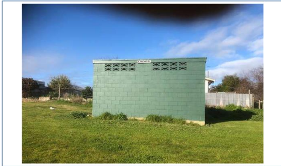
Fig:3&4. Toilet block near Tennis court
