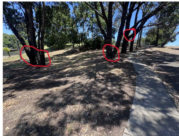
5 trees, dead grass due to trees, multiple cracks showing
