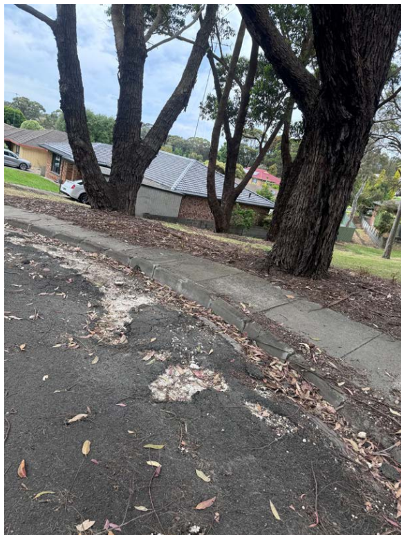
Roadway damaged by tree roots, raised footpath
