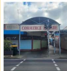
3 Commerce Arcade and Ripley Arcade laneway entrances
