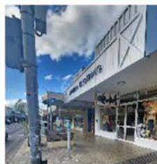
3 Commerce Arcade and Ripley Arcade laneway entrances
