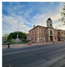
1 Commercial Street West Civic Precinct
