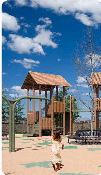
Steel frame tower with recycled timber cladding
