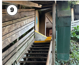
Stairs up from the sinkhole.
