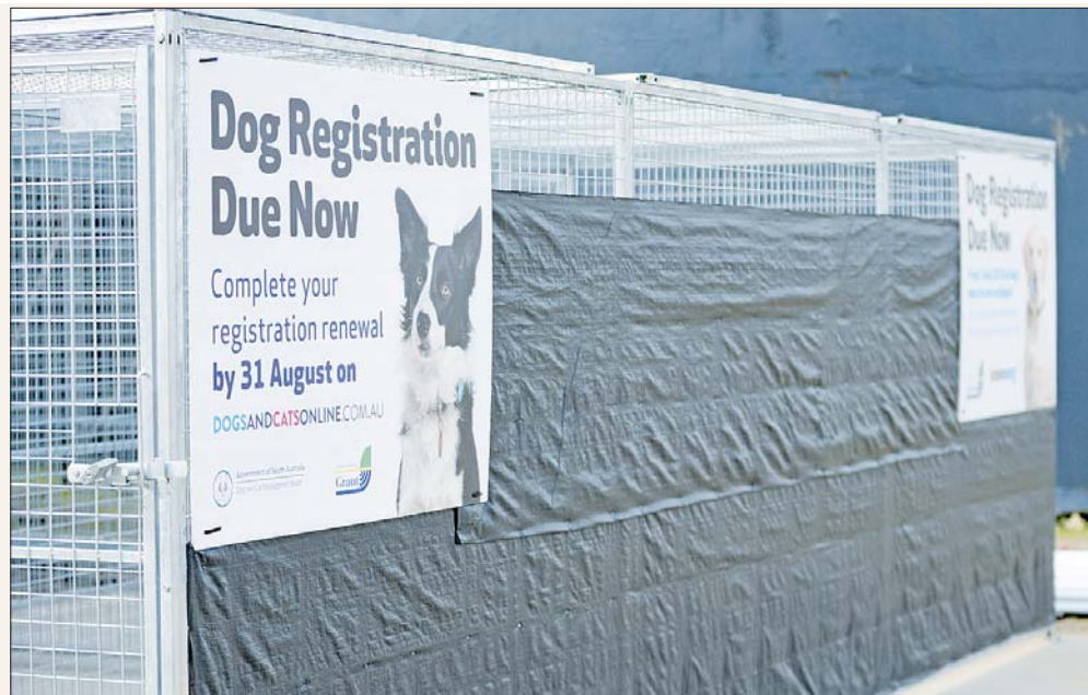
NEW INFRASTRUCTURE: The new dog pound being assembled at the Grant District Council depot.
