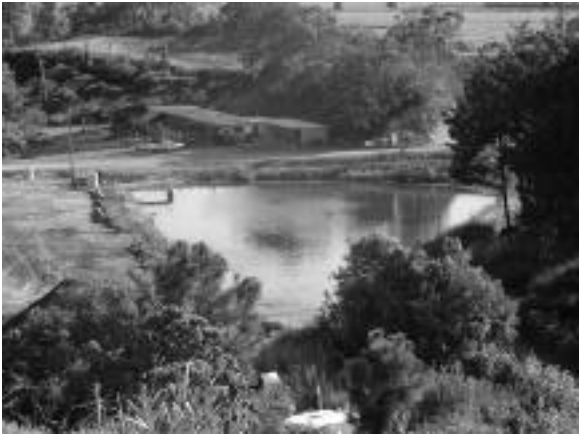
Photo 1 Leachate pond and excess leachate is taken away during high rainfall period
