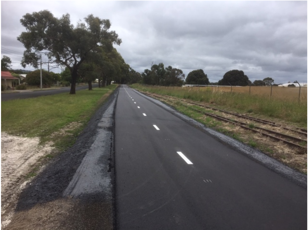
Figure 2: Rail Trail looking West to Pick Ave
