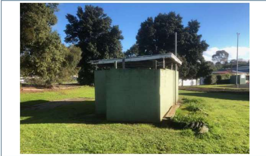
Fig: 1&2. Toilet block near netball court
