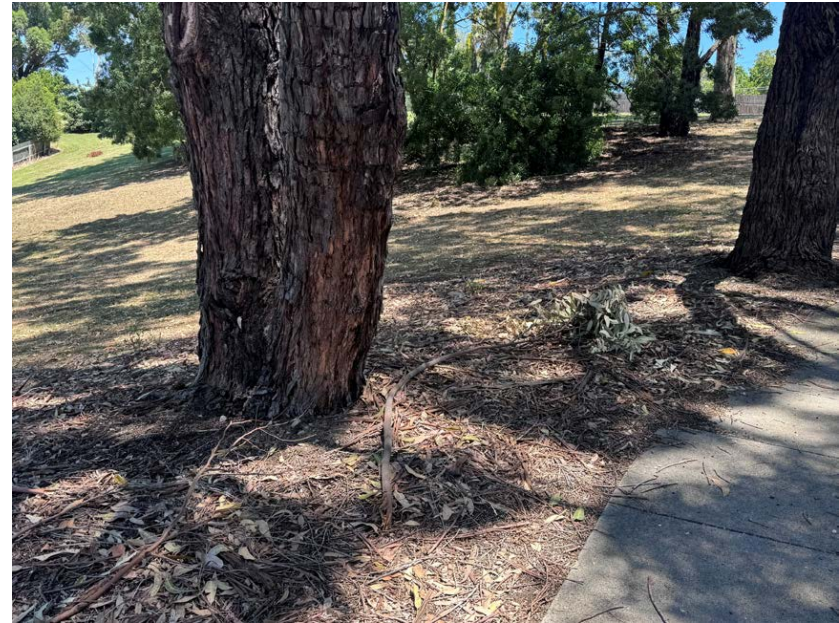
2 trees bordering roadway, small limb, shows distance from footpath
