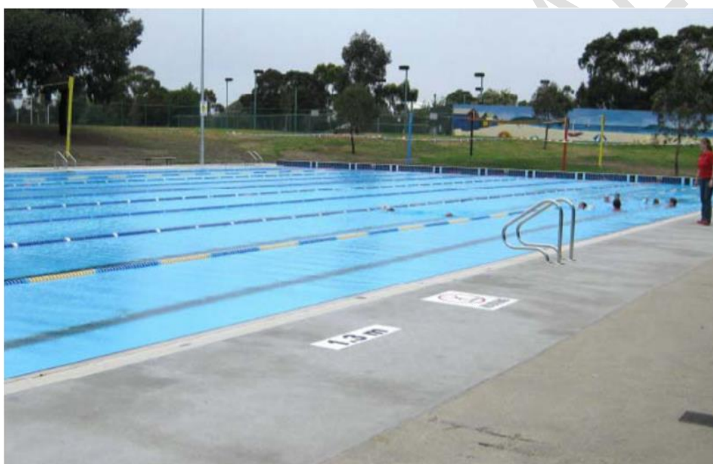
Figure 3: The above image shows the completed pool refurbishment at Northcote Aquatic Centre. Note the two flush wet deck sides and the pediment end walls. The existing 50m pool had a hob to the full perimeter that was removed as part of the refurbishment. At Mount Gambier Aquatic we propose to raise the concourse level to avoid expensive concreting works.
