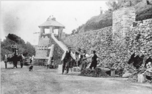
BUILT IN A DAY: Men hard at work during the construction of the Rook Walk on November 27, 1918. A public holiday was declared in Mount Gambier to allow 800 men to build the walkway. The walkway, a 10ft stone wall and three lookouts were completed in one day.
