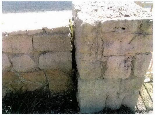
6. Disengagement of pier at extreme east end of the wall (E end of 4.5m long section)
