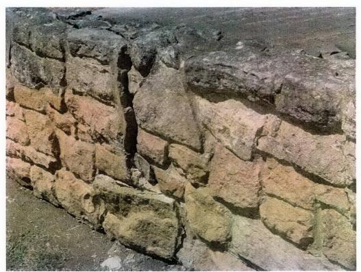
8. Longitudinal crack in photo 7 extends to severely displaced vertical crack
