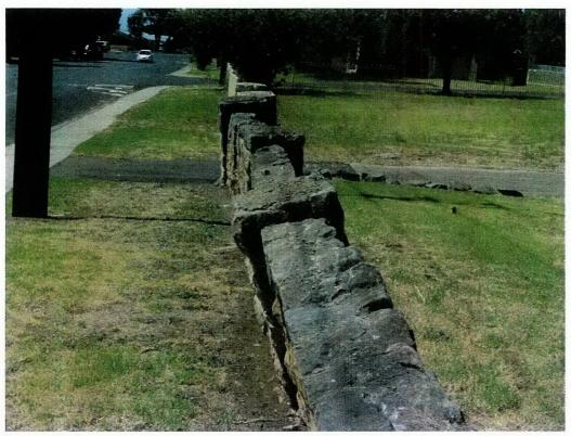
5. Rotation / lateral displacement of wall, looking from near the middle towards the east end
