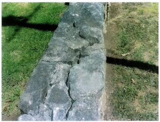
7. 20mm wide longitudinal crack near east end of wall, 2m west of the driveway
