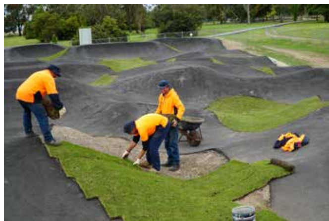
Pump Track construction at Hastings Cunningham Reserve.
