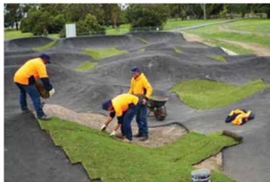
Pump Track construction at Hastings Cunningham Reserve.
