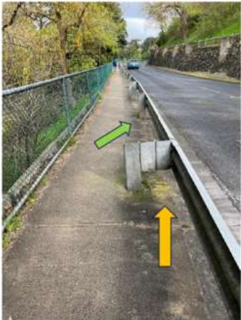
Example of vehicle barrier on the Kingston Bridge in the Riverland, SA. This type of barrier takes up less room, provides protection for trail users, provides more space and allows for improved pedestrian and bicycle access.
