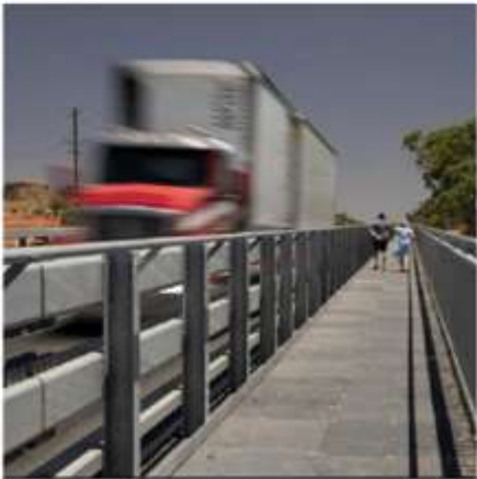
Example of vehicle barrier on the Kingston Bridge in the Riverland, SA. This type of barrier takes up less room, provides protection for trail users, provides more space and allows for improved pedestrian and bicycle access.
