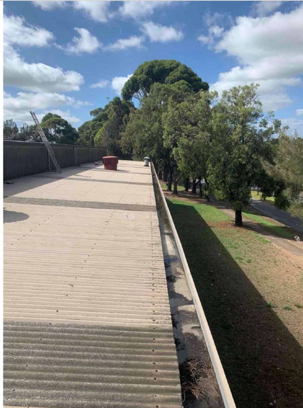
Photo shows the main shed box gutter full of council property gum leaves at the eastern end of the dwelling. Zoom in photos to see how full the box gutter is.
