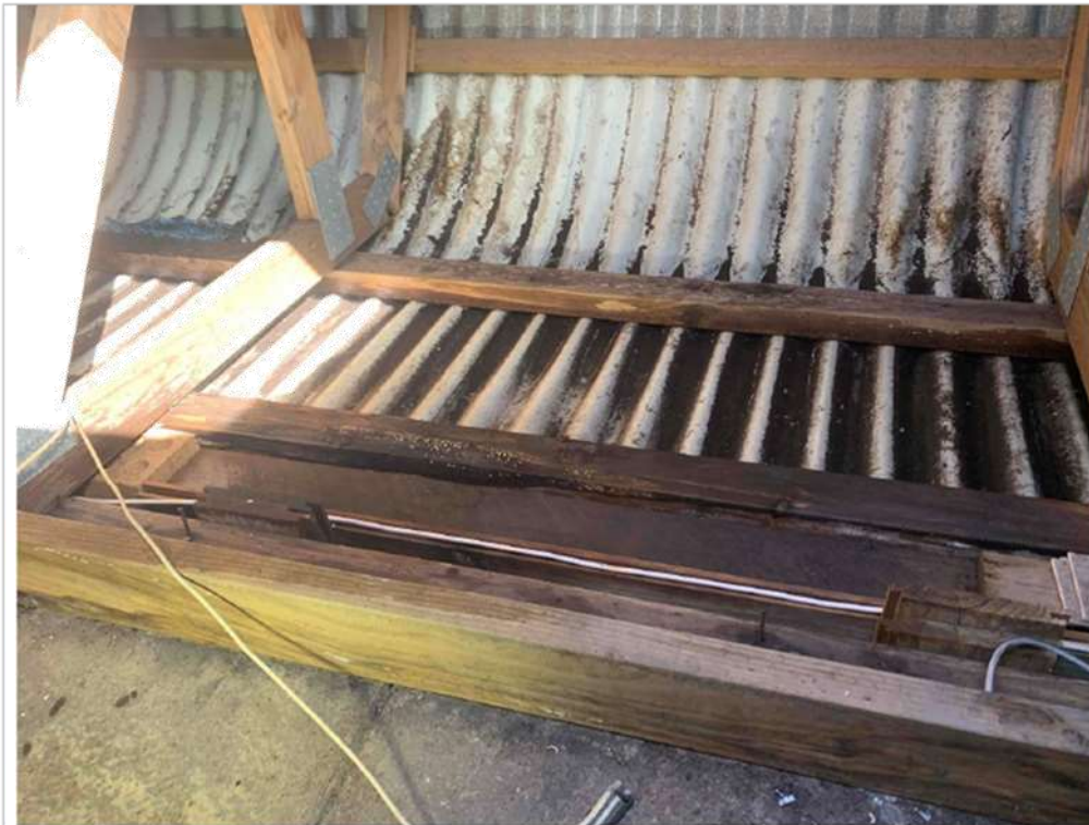
Photo shows an internal view of the roof flashing showing all timber work wet from blocked gutters full of boundary gum tree leaves clogging up the office guttering
