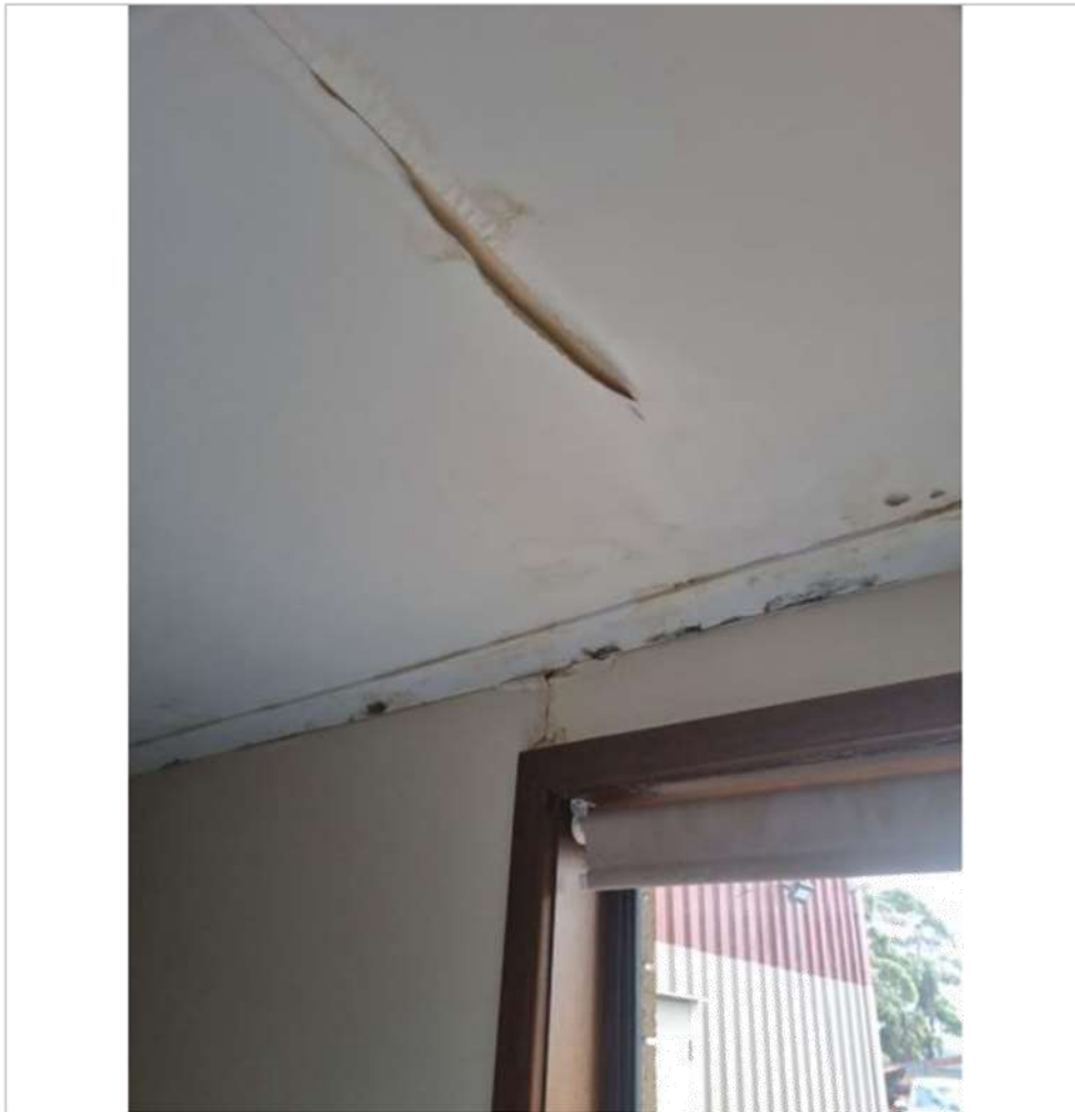
Photo shows the water damage to the ceiling space in the SAPOL office
