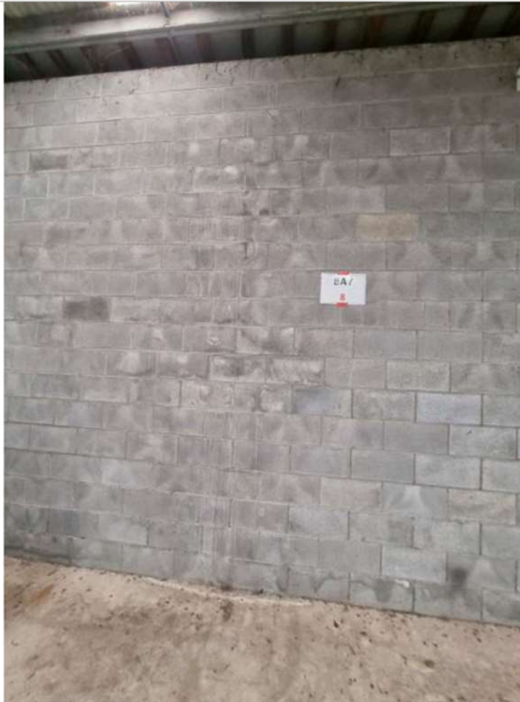
Photo shows internal main shed wall water damage from water running over the box gutter and water running down the internal walls of the main storage shed.
