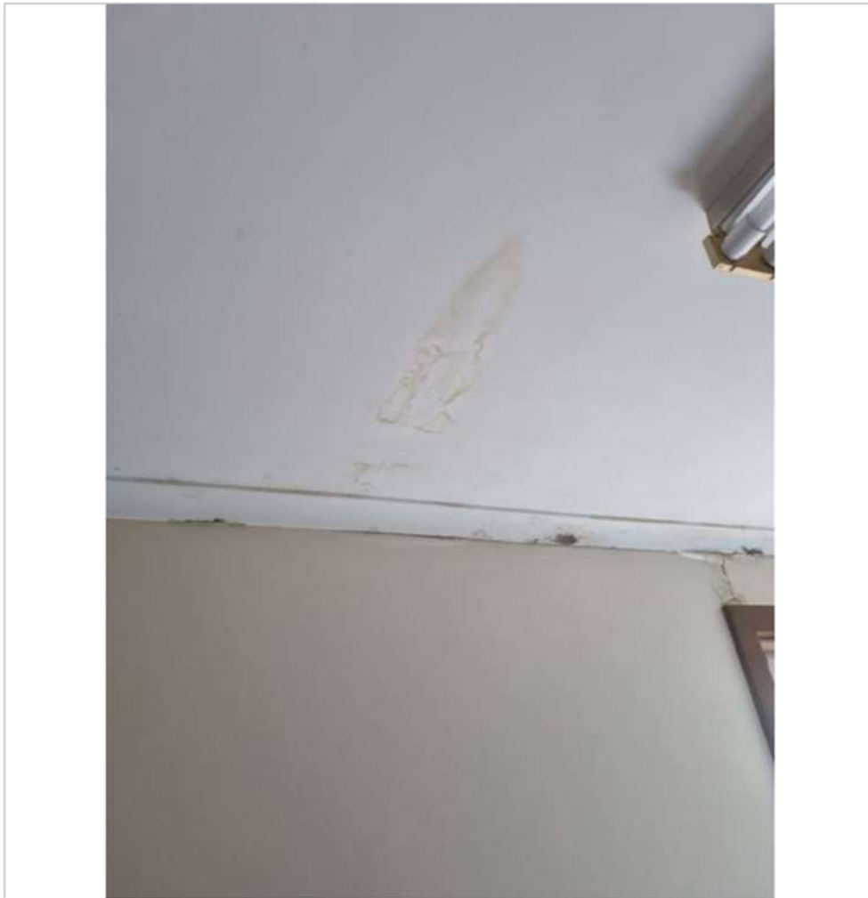
Photo shows water damage to internal office ceiling.
