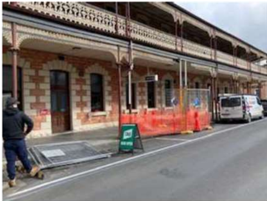
Location of Acro Props – Previously damaged balcony posts
