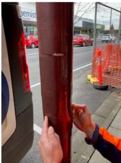
Additional Balcony post with fracture
