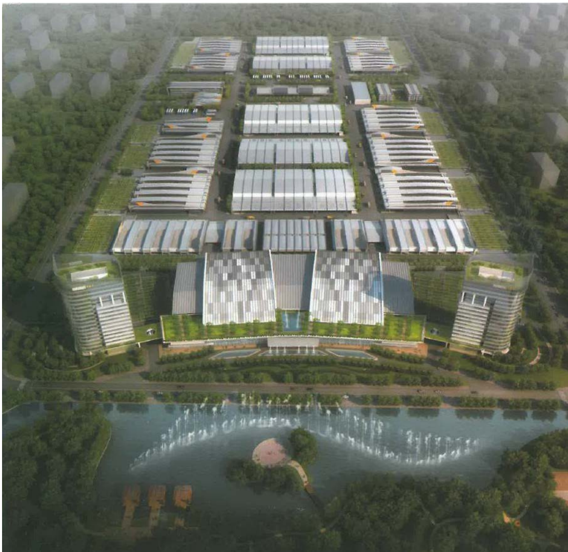
Keppel International Coldchain Logistics Park
