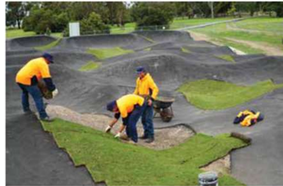
Pump Track construction at Hastings Cunningham Reserve.
