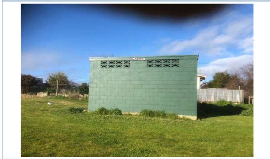
Fig:3&4. Toilet block near Tennis court
