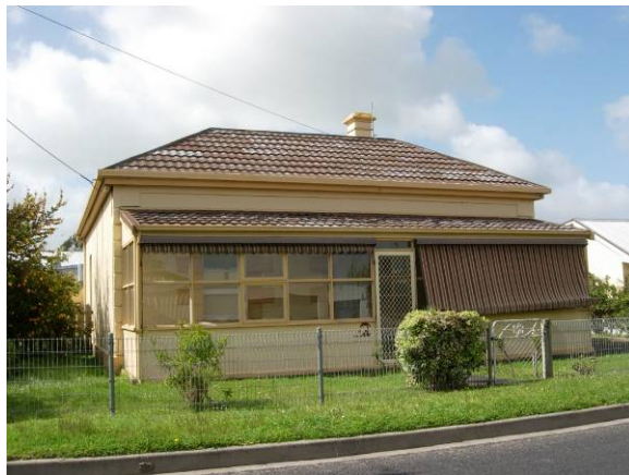
House, 4 Gerloff Street
