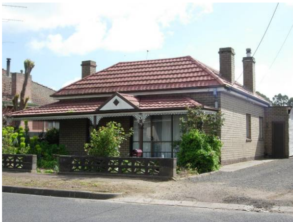
House, 5 John Street
