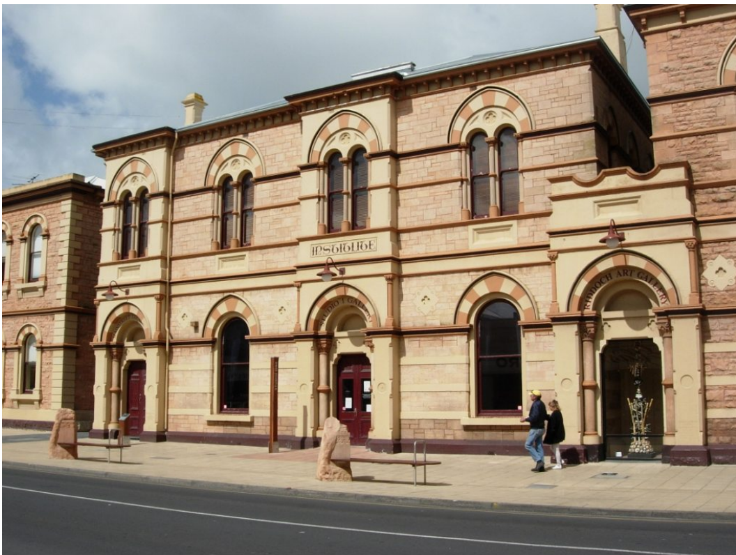
View of the former Mount Gambier Institute
