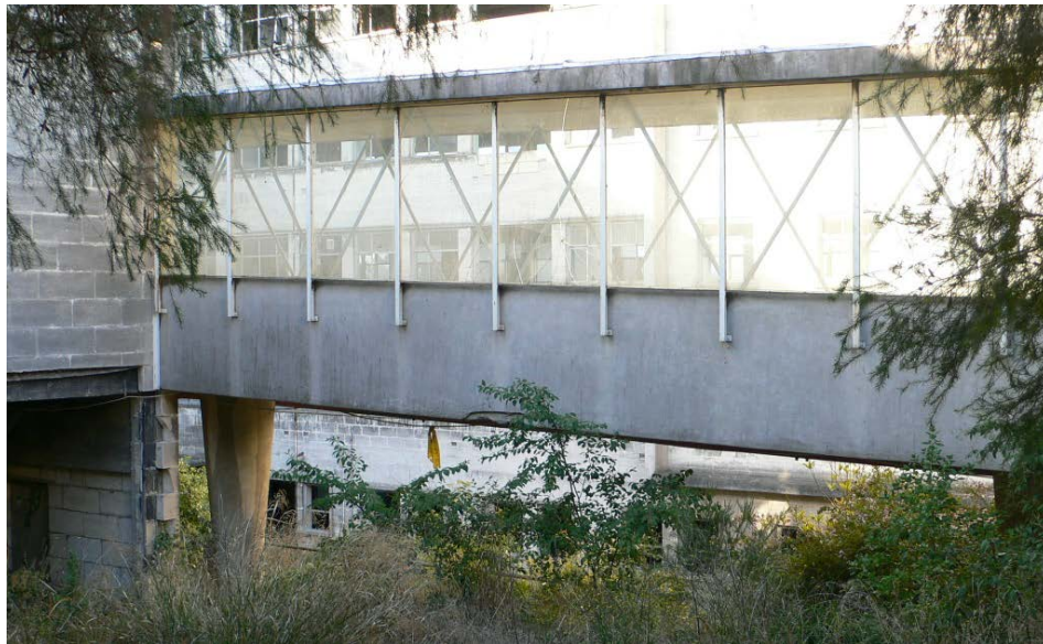
Linking elevated Walkway from main building to Nurses' Home
