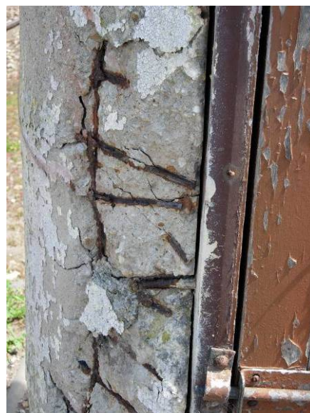
Views of corroding metal reinforcing
