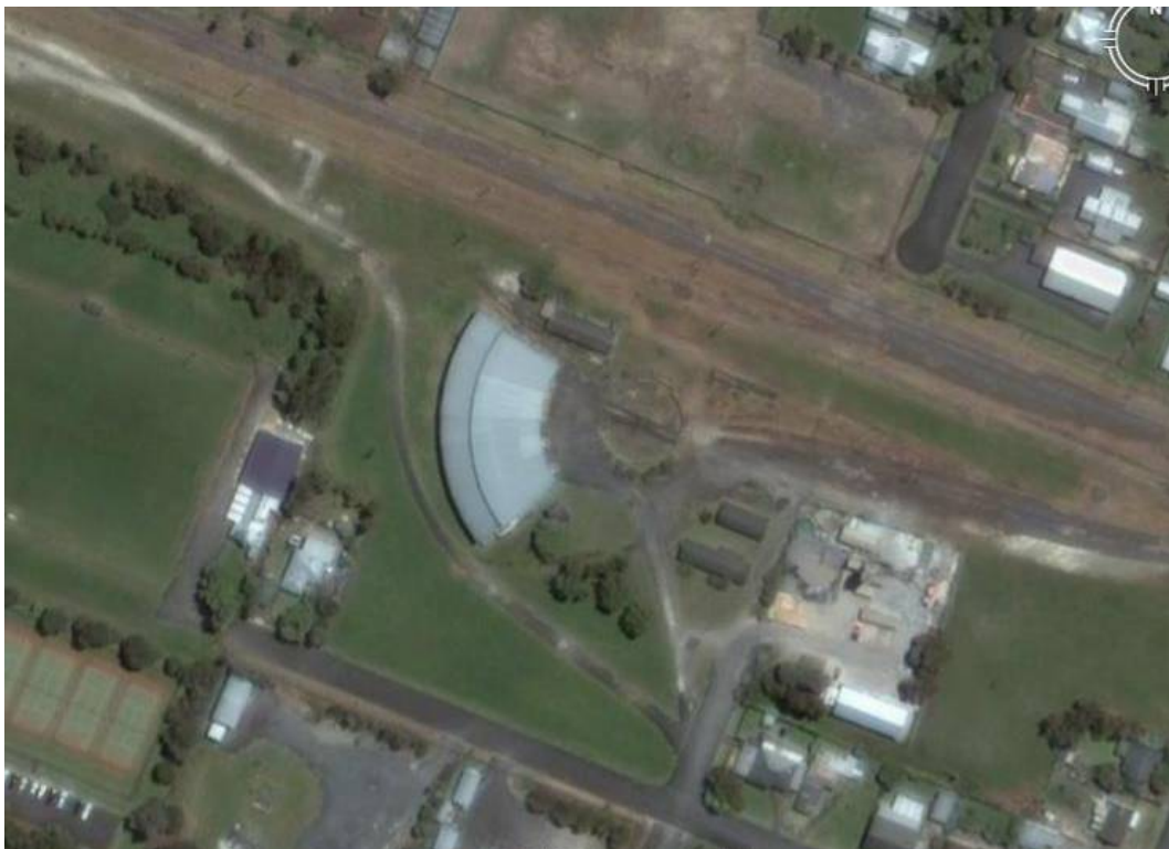
Aerial view of turntable showing segmental form of round house
