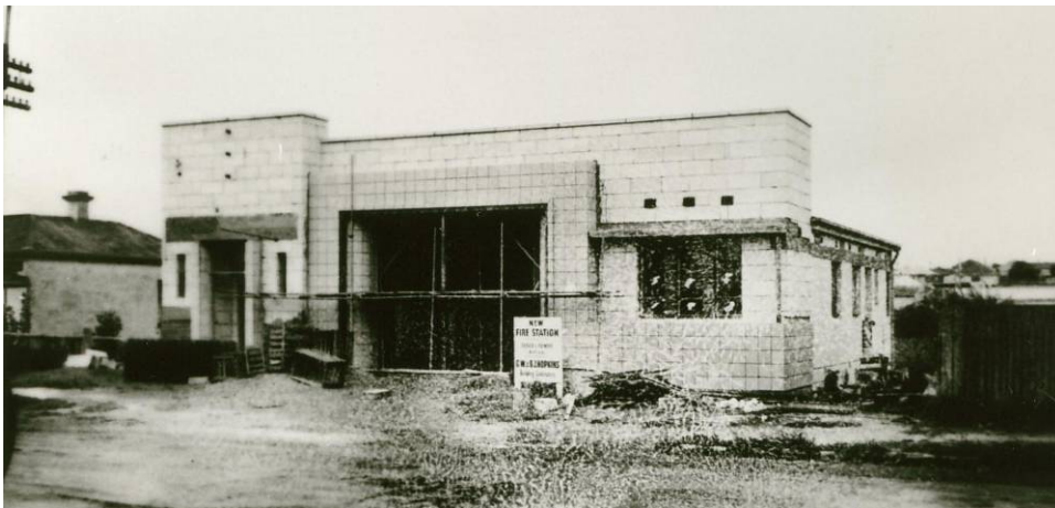
Mount Gambier Fire Station under construction, 1956 (Source: Les Hill Collection)
