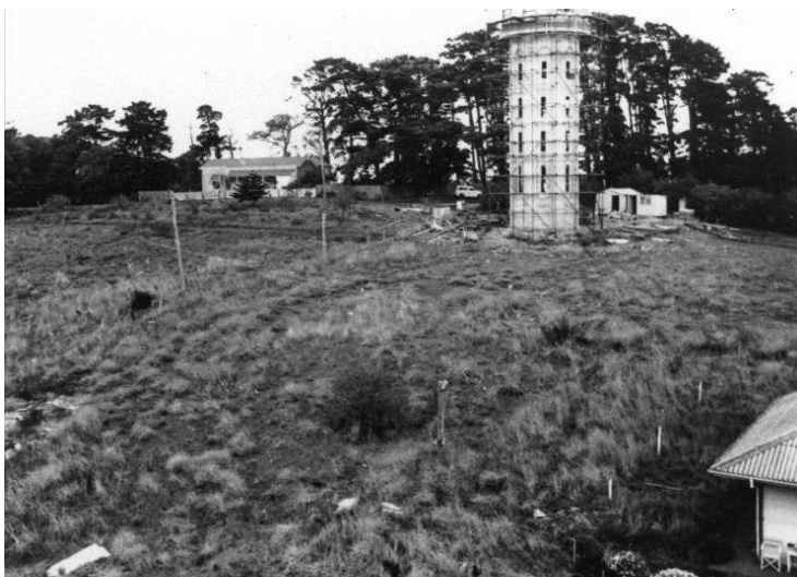
View of water tower during construction, 1959
