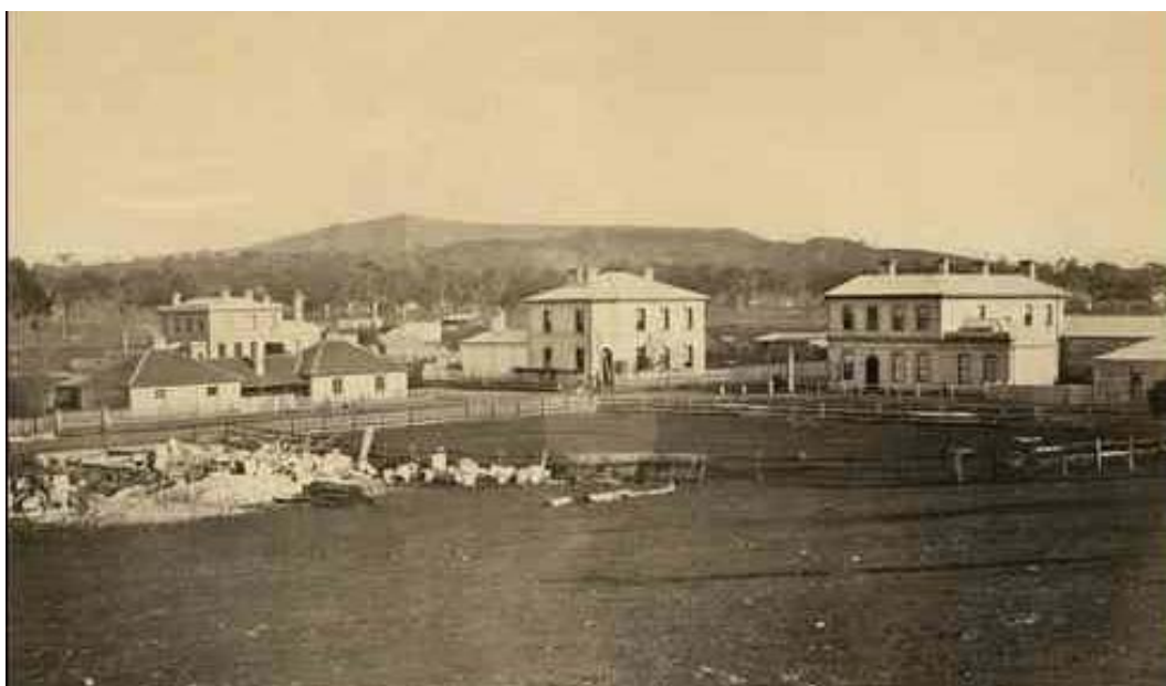
The intersection of Commercial Street and Penola/Bay Roads with the Telegraph Station, Bank and Mount Gambier Hotel, c1863 (Source: State Library of South Australia, B3076)
