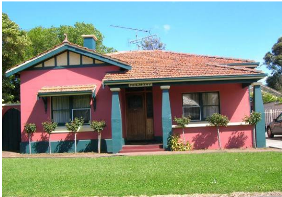
House, 10 Anzac Street
