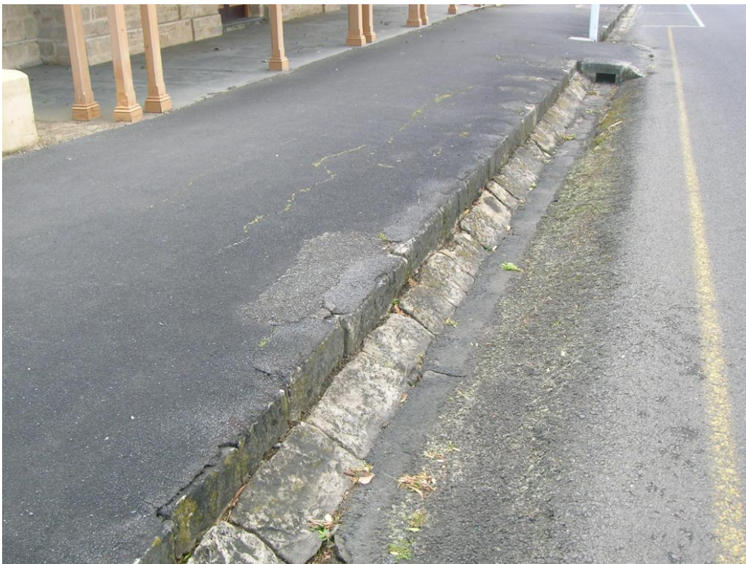
Views of the dolomite kerbing at 42 Bay Road, Mount Gambier
