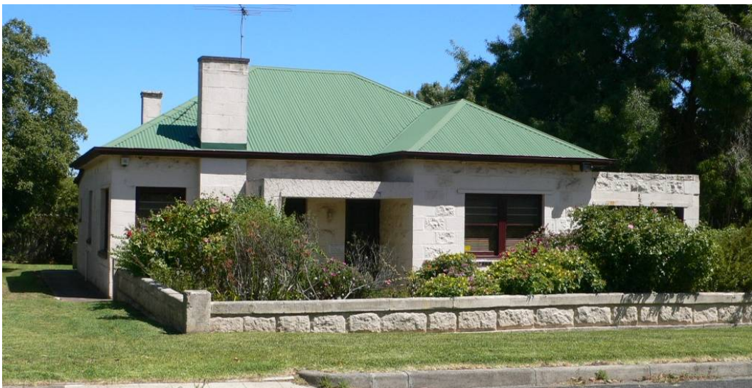
Power Street (house 1940s)
