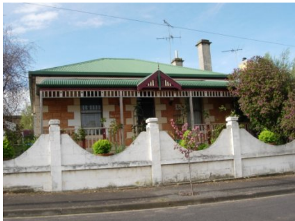
House, 4 Agnes Street
