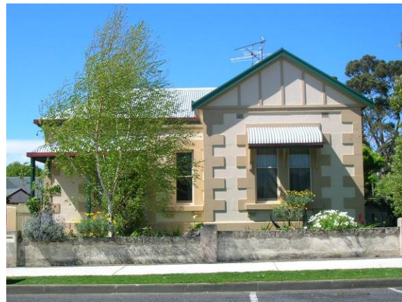
House, 45 Ferrers Street
