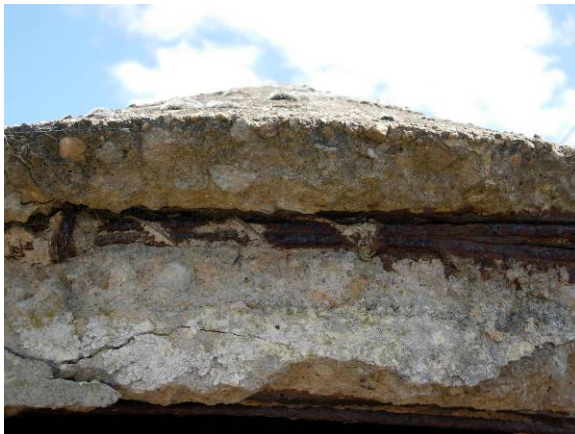
Views of corroding metal reinforcing
