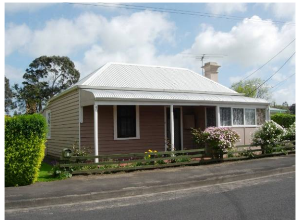
House, 5 Gerloff Street
