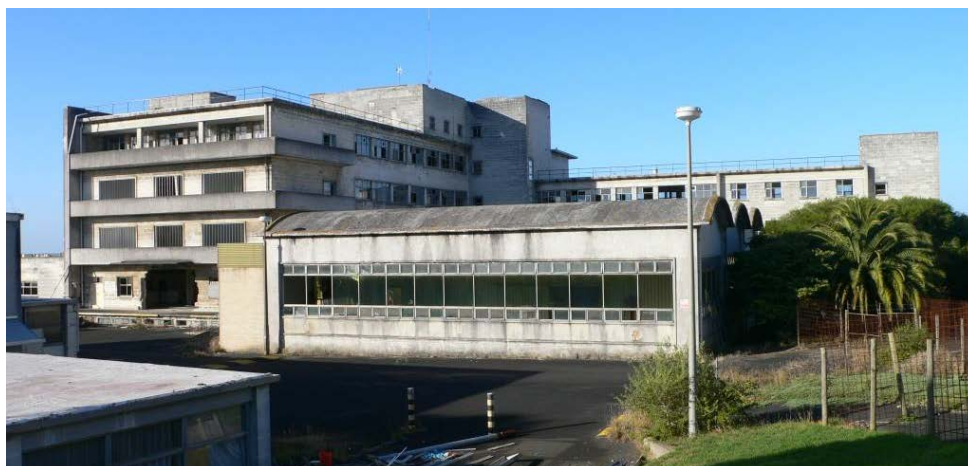
View of Hospital buildings from south – showing laboratories and parabolic roof forms
