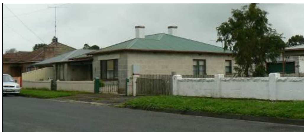
Photos 2 & 3: Younger Dwellings have varied setbacks, roof forms, pitches and materials
