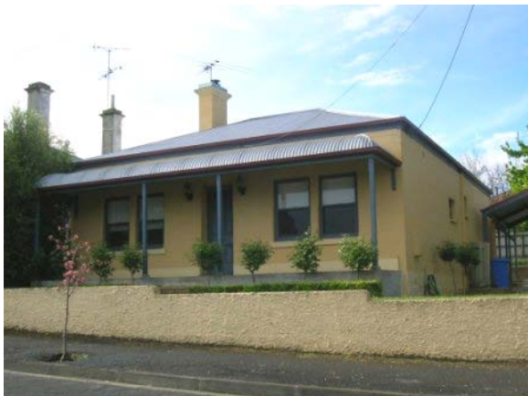
House, 2 Agnes Street
